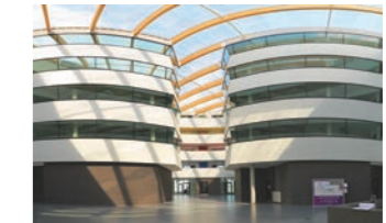
Chobham Academy. Renovation of the 2012 Olympics security control centre structure into an all-age academy for a newly formed residential community.
