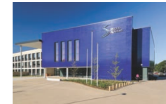
Strood Academy. State-of-the-art development to transform poor-performing schools, with a focus on renewable energy.
