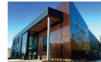
Hessle High School. A new-build secondary school, plus refurbished listed building. Located in East Yorkshire, it is part of The Consortium Academy Trust.
