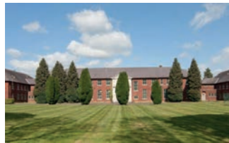
Heyford Park Free School. Split campus on recommissioned RAF site, plus refurbishment of a Cold War era sports facility to provide specialist teaching spaces.
