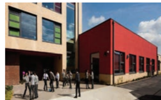
Priestmead Primary. Redevelopment for the largest primary school in the UK, involving phased demolition and a new-build primary and nursery.
