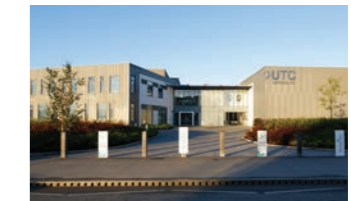
Oxfordshire UTC. A new-build specialist STEM college in Didcot on a two-hectare greenfield site, which blends academia and vocational training.
