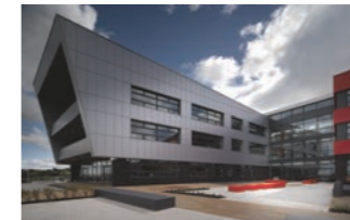
Blackburn Central High. The amalgamation of three existing schools into one. The vast building has 80% of its heating needs met by a biomass boiler.
