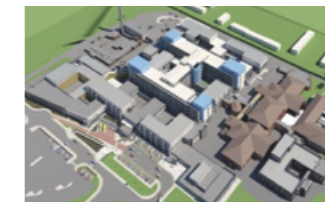
Prince Charles Hospital, Merthyr Tydfil. The phased refurbishment of an existing 40-year-old district general hospital.
