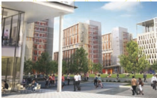
Wood Lane Studios. Imperial West. The first completed building for Imperial College London's new campus, it features 606 postgraduate student rooms alongside nine key worker flats.
