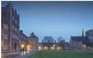
Jesus College. University of Cambridge. The refurbishment of the Grade II development resulted in an estimated 45 percent less energy usage, and significantly reduced the building's carbon footprint.
