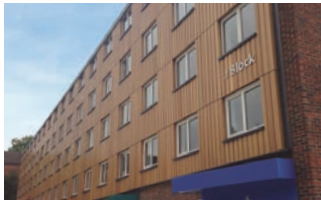
Glen Eyre Block J. University of Southampton. A refurbishment project with 87 bedrooms, enhanced common areas, and campus reception. It will be used as a benchmark for future refurbishment projects.
