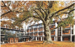
Kendrew Quadrangle. St John's College. Top-class accommodation for 68 students and six junior research fellows, along with communal spaces, café, and gym.
