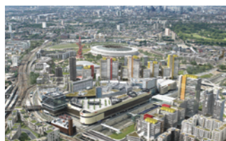
International Quarter. Prime office space with the highest sustainability standards in East London's Stratford City.
