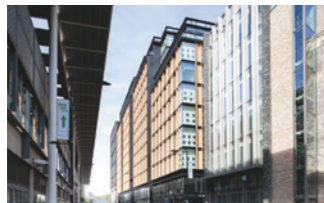
6 St Pancras Square. High-spec offices on the vibrant King's Cross redevelopment site, occupied by Google.
