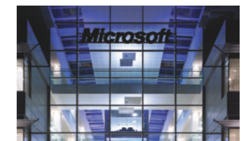
Microsoft Building 5. Award-winning headquarters for 700 staff in a flexible, contemporary environment.
