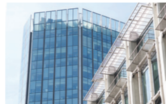
125 Old Broad Street. Twenty-six-storey tower redevelopment in the heart of London's financial district.
