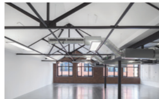
Concordia Works. Award-winning unique loft-style workspace in Leeds city centre with future-proofed services.
